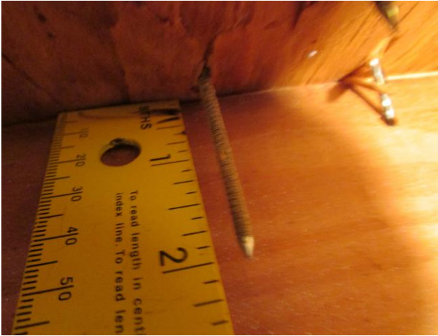
Roof Deck Attachments: 8d nails @ max. 6"
