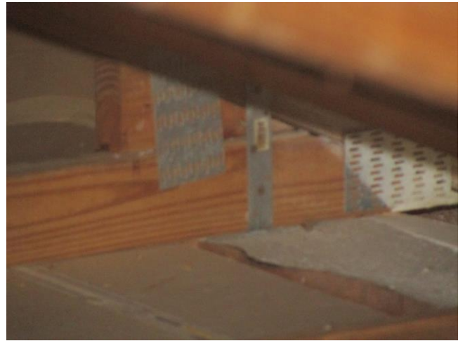
Roof Wall Attachments: Wraps with 3 nails
