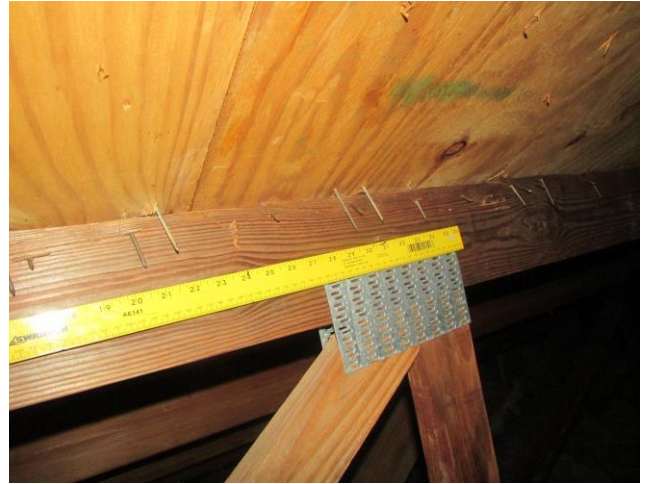
Roof Deck Attachments: 8d nails @ max. 6"
