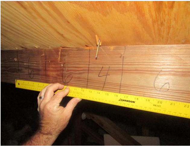
Roof Deck Attachments: 8d nails @ max. 6"
