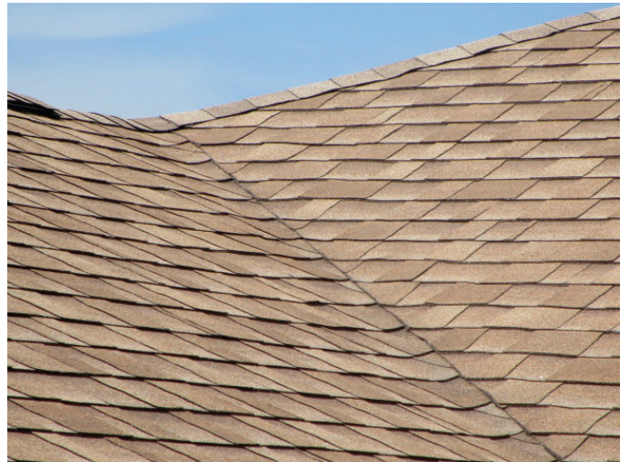
2006 dimensional asphalt shingle "other" style roof
