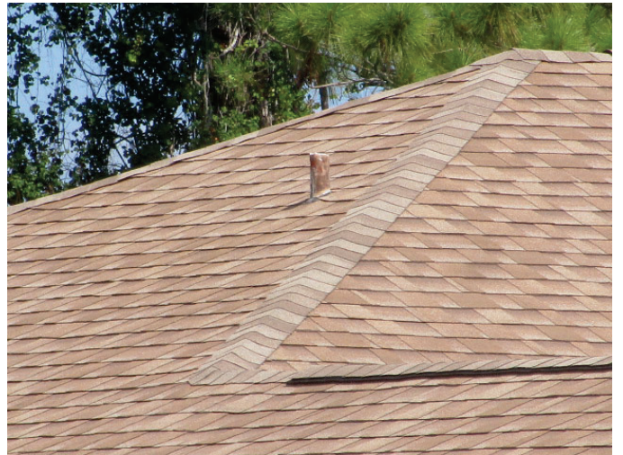
2006 dimensional asphalt shingle "other" style roof
