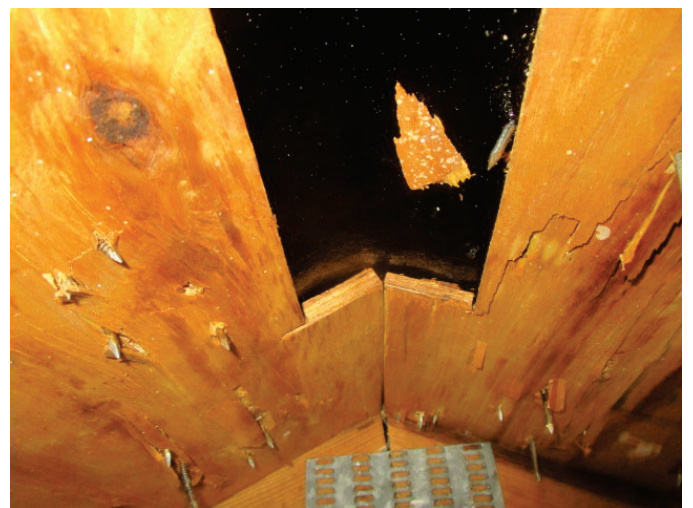
secondary water barrier as viewed from the attic
