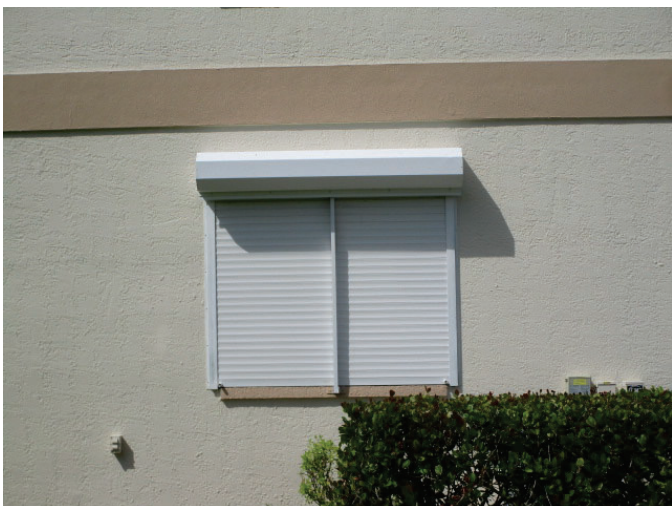
non impact windows- some w/protection
