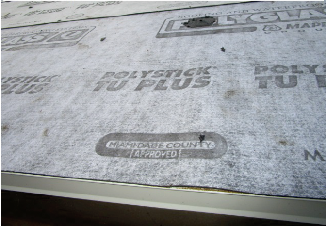
#6) secondary water barrier
