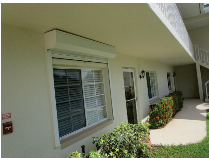
non impact windows- some w/protection
