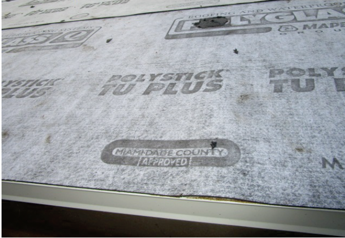
#6) secondary water barrier
