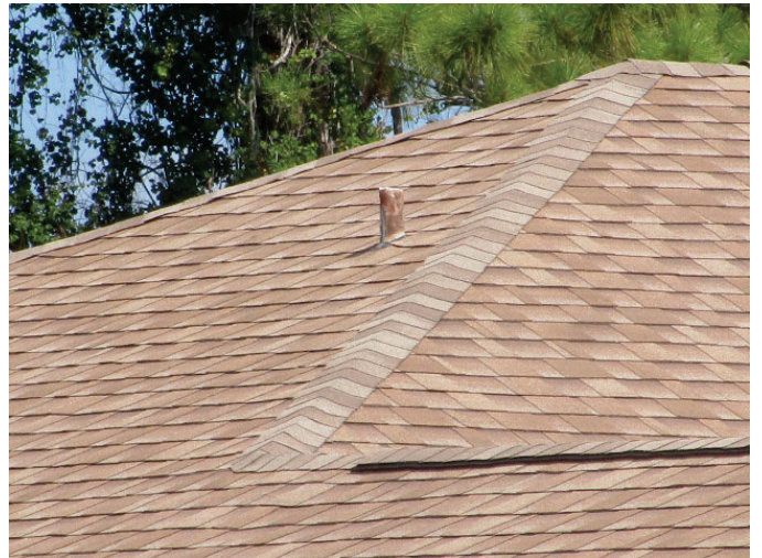
2006 dimensional asphalt shingle "other" style roof
