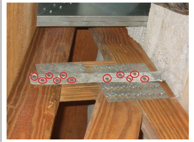
ROOF TO WALL ATTACHMENT – Properly installed Clips
