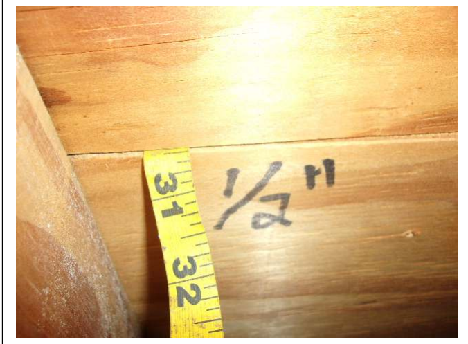
ROOF DECK THICKNESS – ½ inch plywood
