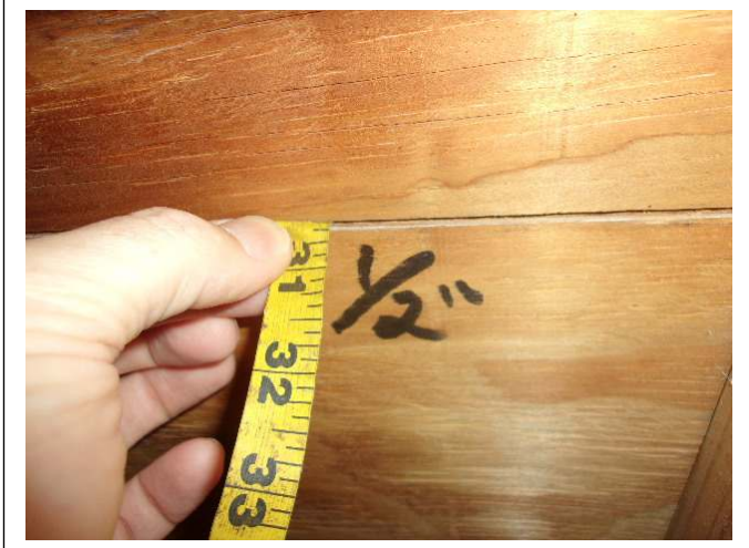
ROOF DECK THICKNESS – ½ inch plywood
