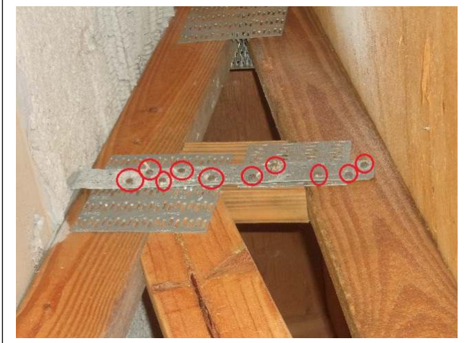
ROOF TO WALL ATTACHMENT – Properly installed Clips
