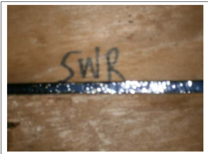
SECONDARY WATER BARRIER – A polymer adhesive (peel & stick) SWR Barrier was installed on the entire roof deck in 2022
