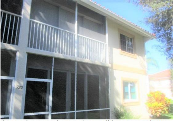
#7) opening protection: non impact sliders some w/shutters
