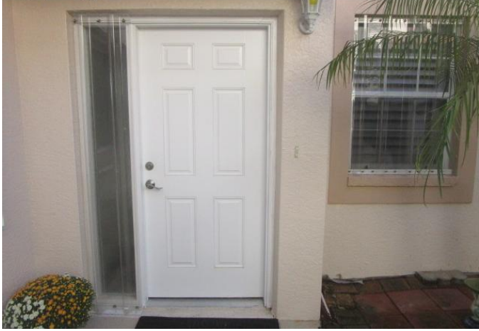
#7) opening protection: metal clad doors (some w/protection)
