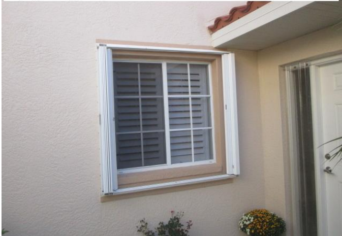
#7) opening protection: some windows have shutters
