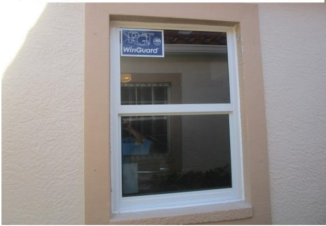
#7) opening protection: some windows are impact rated
