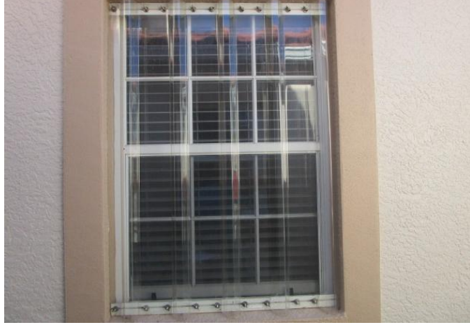
#7) opening protection: some windows have shutters
