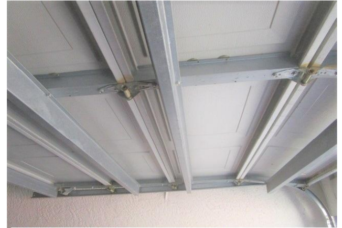
#7) opening protection: non impact garage doors
