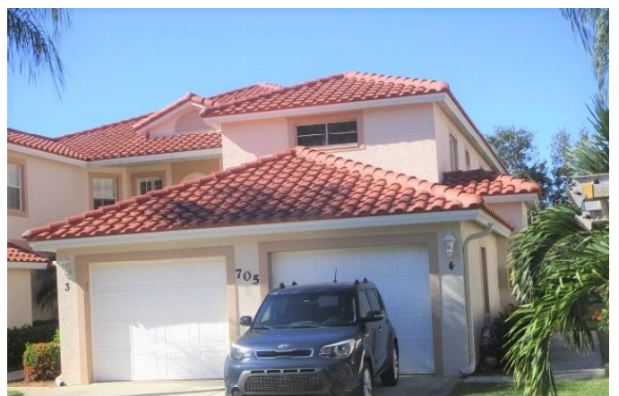
#5) roof geometry: HIP style roof **wall type construction: 100% reinforced masonry
