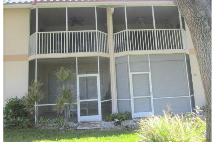
#7) opening protection: non impact rear sliders (some w/shutters)
