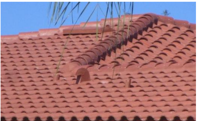
#2) roof covering: 2021 TILE HIP style roof PRBD2021-0419301 applied 4/27/2021
