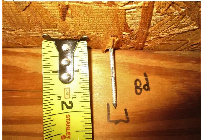
#3) roof deck attachment: 8d nails
