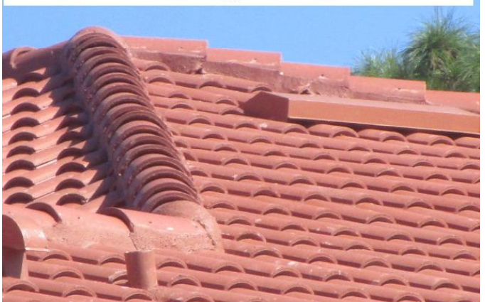
#2) roof covering: 2021 TILE HIP style roof PRBD2021-0419298 applied 4/27/2021
