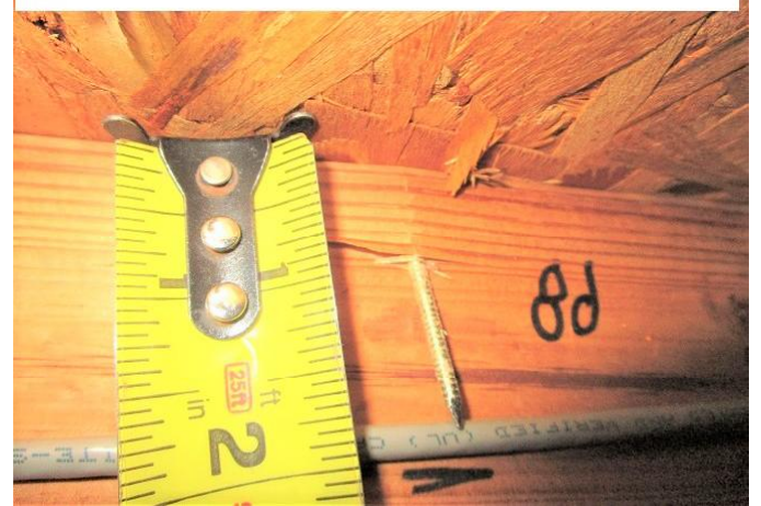
#3) roof deck attachment: 8d nails
