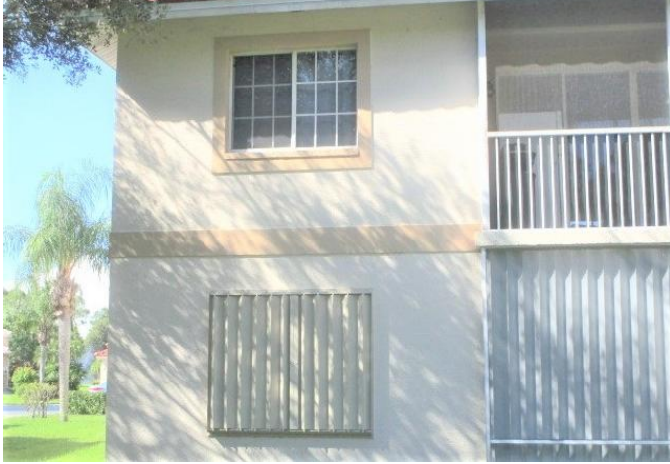
#7) opening protection: non impact windows (some w/protection)
