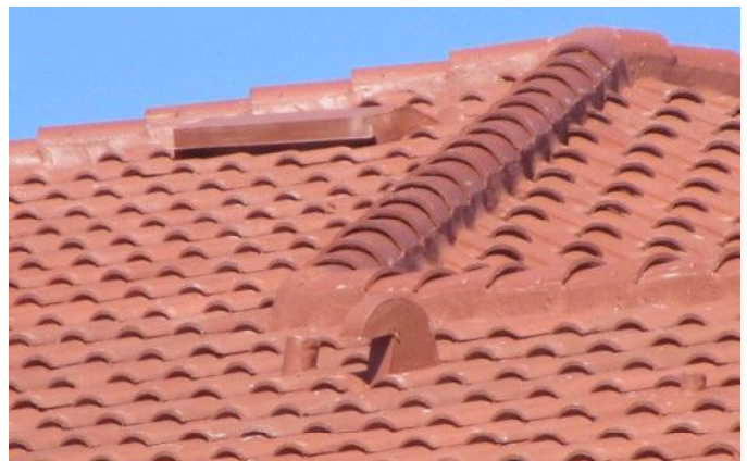
#2) roof covering: 2021 TILE HIP style roof PRBD2021-0419295 applied 4/27/2021
