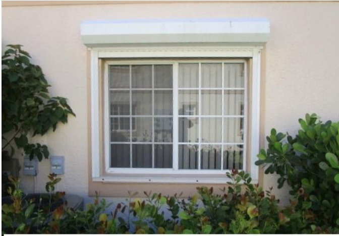
#7) opening protection: non impact windows (some w/shutters)
