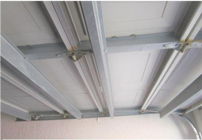
#7) opening protection: non impact garage doors
