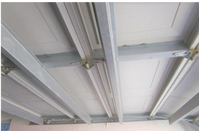
#7) opening protection: non impact garage doors
