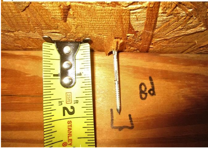
#3) roof deck attachment: 8d nails
