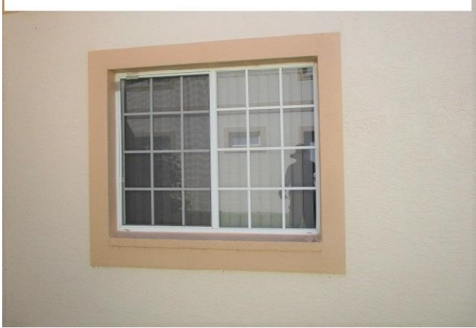
#7) opening protection: non impact windows
