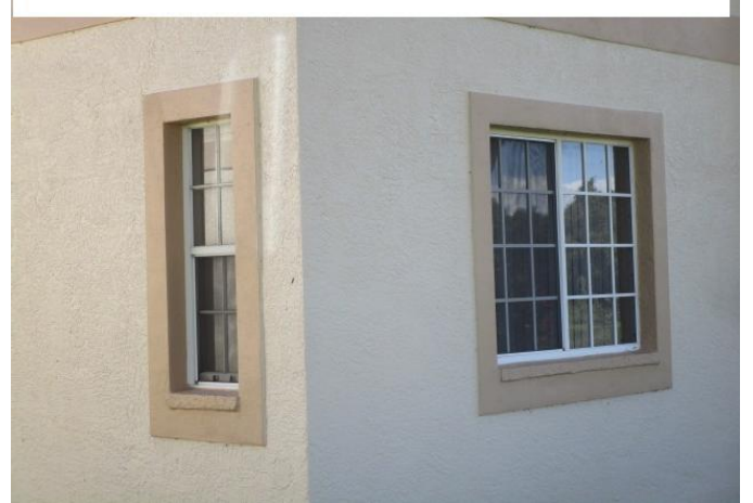
#7) opening protection: non impact windows
