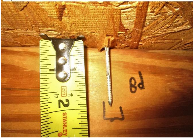
#3) roof deck attachment: 8d nails
