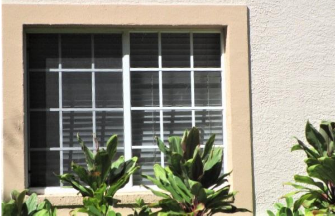
#7) opening protection: non impact windows
