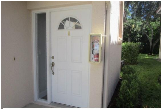
#7) opening protection: non impact front entrance
