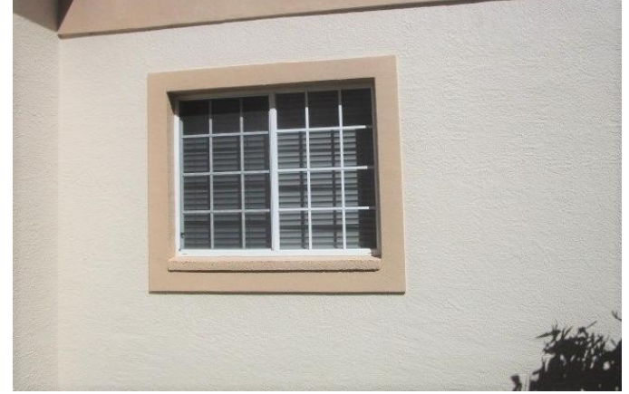
#7) opening protection: non impact windows
