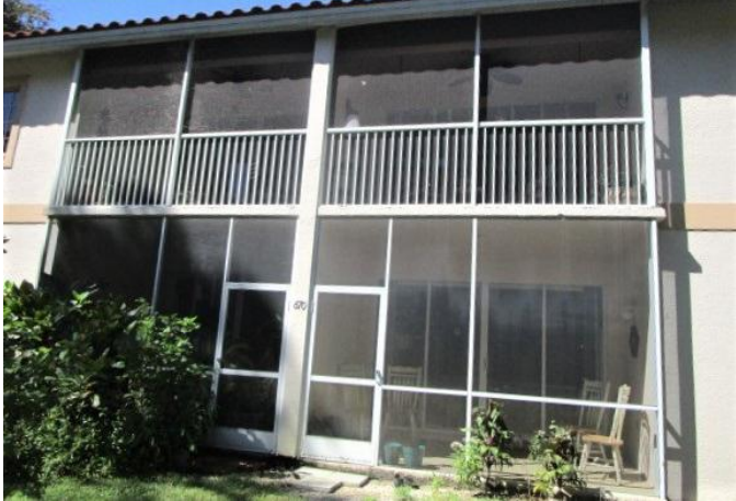
#7) opening protection: non impact rear sliders
