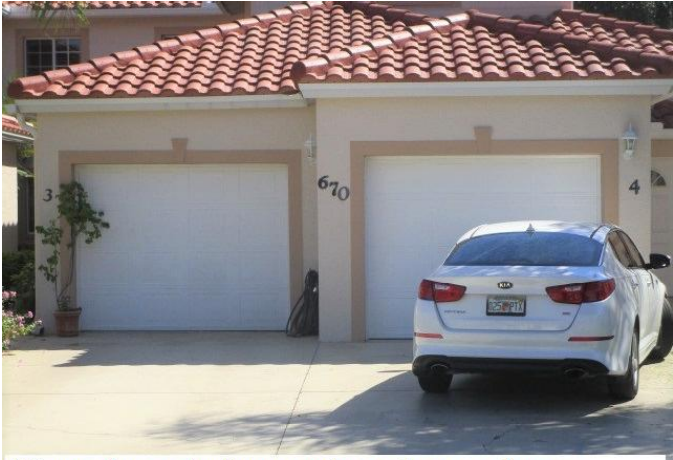
#7) opening protection: non impact garage doors
