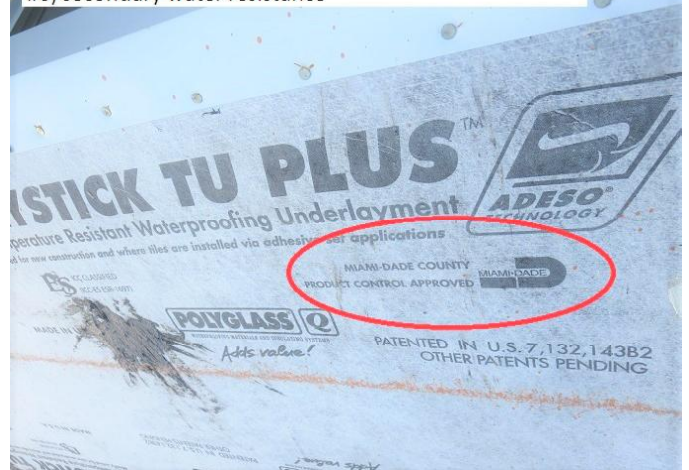
#6) secondary water resistance
