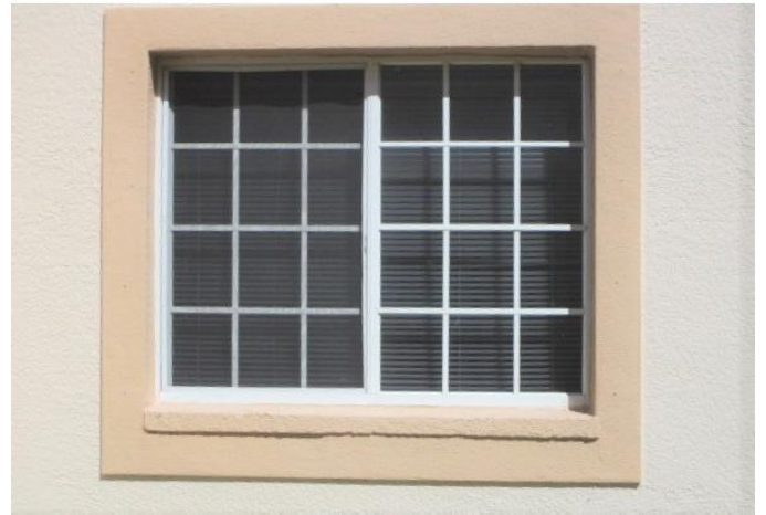
#7) opening protection: non impact windows (some w/protection)
