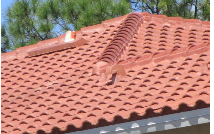
#2) roof covering: 2021 TILE HIP style roof PRBD2021-0419286 applied 4/27/2021
