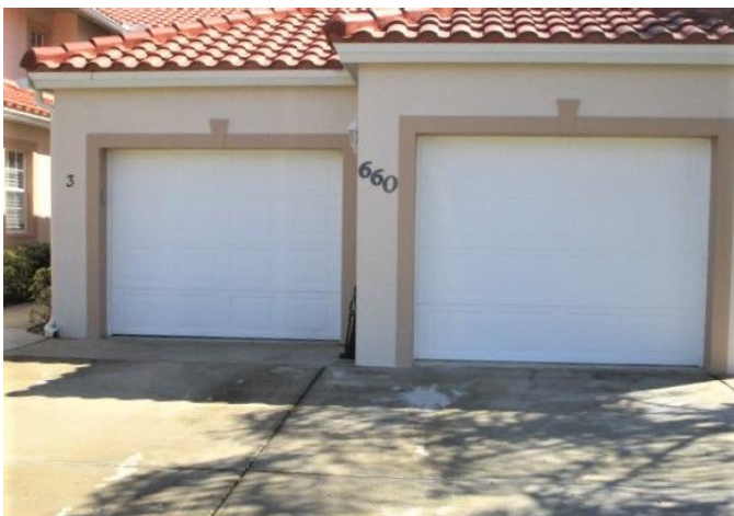
#7) opening protection: wind rated non impact garage doors
