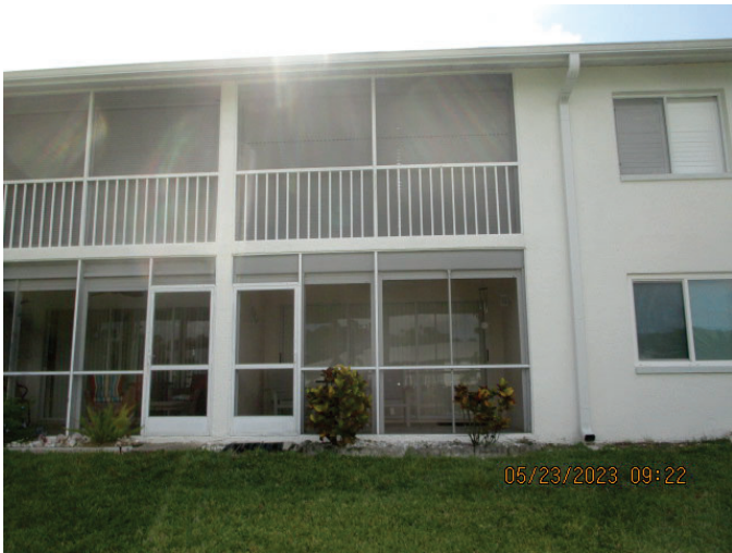
rear porches- non impact sliders- some w roll down shutters
