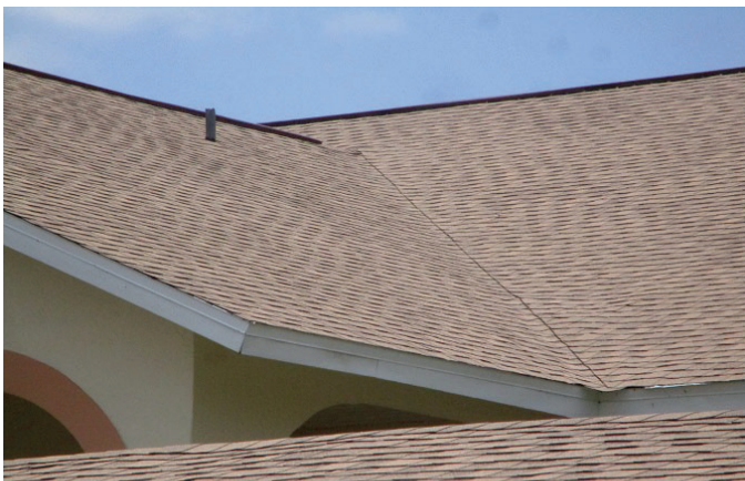
#2) roof covering: 2018 dimensional asphalt shingle "other" style roof PRBD2018-0210028 issued 2/14/2018
