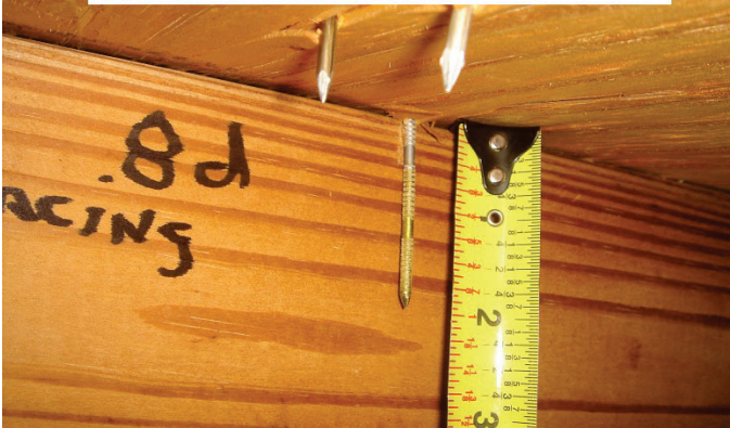
#3) roof deck attachment: 8d nails
