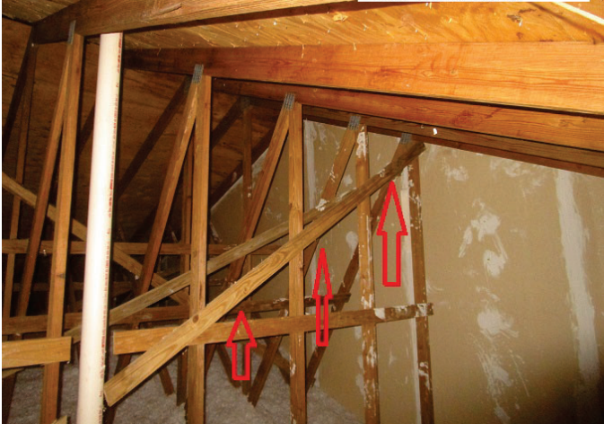
Gable end bracing
