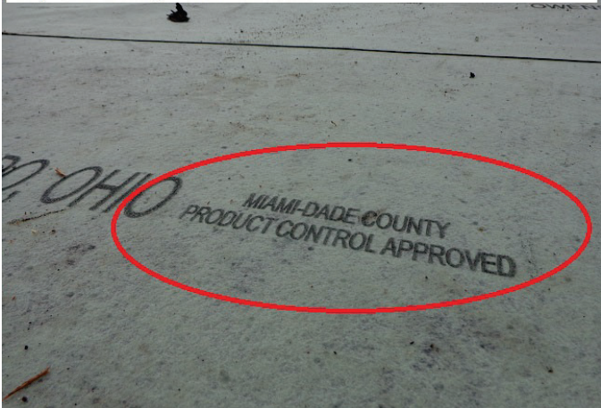
#6) secondary water barrier
