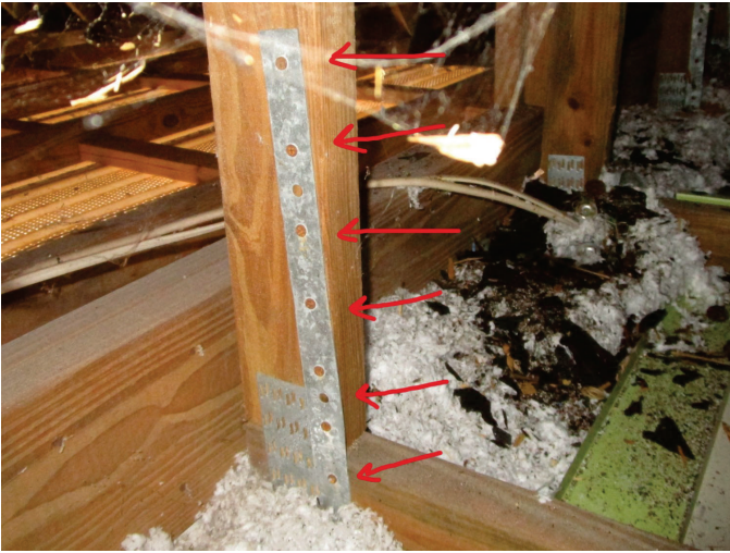
roof to wall attachment: hurricane clips
