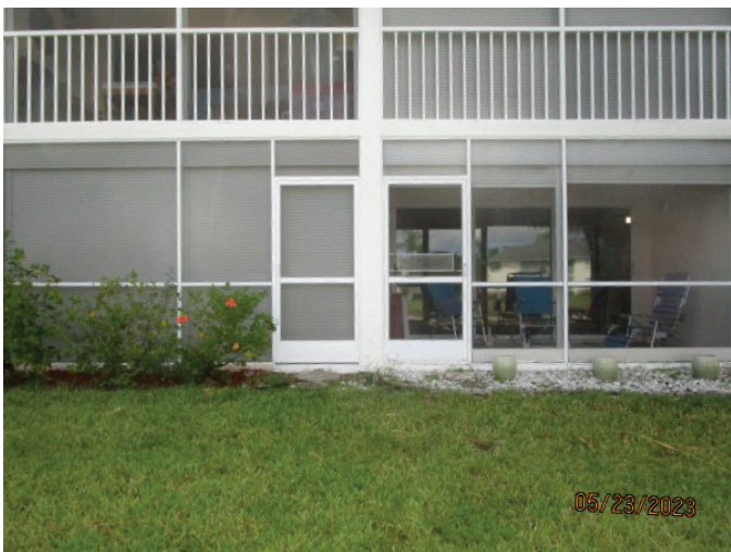
some rear porches have roll down shutters
