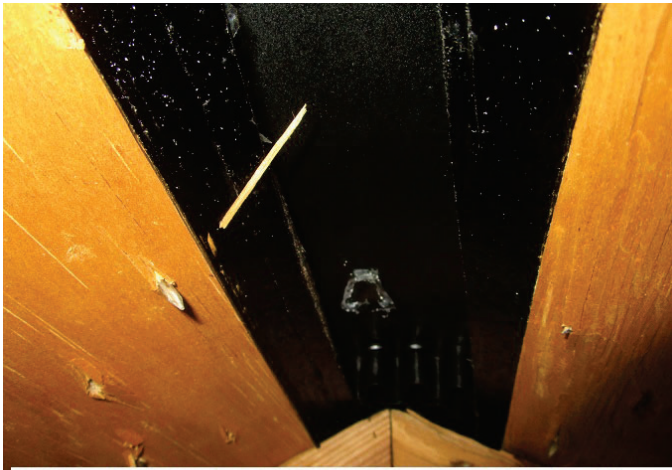
#6) Secondary water barrier/resistance as viewed from the attic
