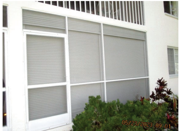
some rear porches have roll down shutters
