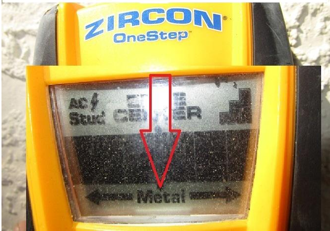
**wall type ocstruction: 85% reinforced masonry
