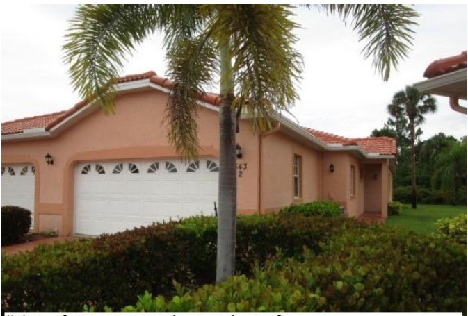
#5) roof geometry: "other" style roof **wall type ocnstruction: 85% reinforced masonry
