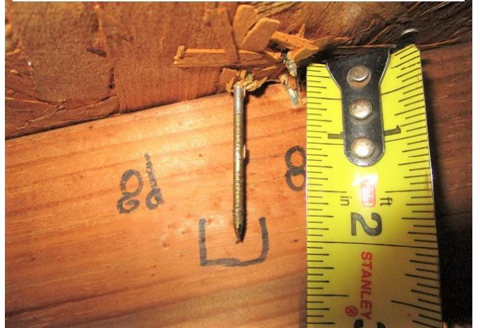
#3) roof deck attachment: 8d nails
