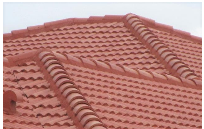
#2) roof covering: 2020 TILE HIP style roof PRBD2020-0731297 applied 7/31/2020
