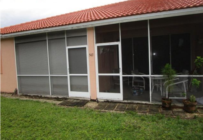
#7) opening protection: non impact rear sliders (1 w/shutters)
