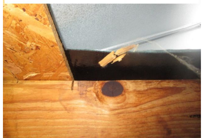
#6) secondary water barrier as viewed from the attic
