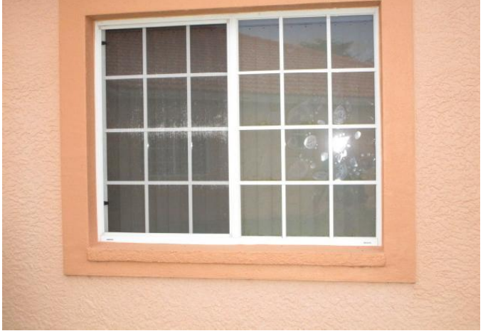
#7) opening protection: non impact windows
