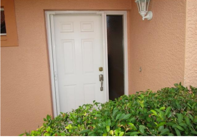
#7) opening protection: metal clad door w/non impact sidelites
