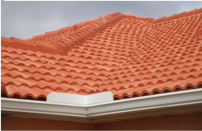
#2) roof covering: 2020 TILE "other" style roof PRBD2020-0731294 applied 7/31/2020
