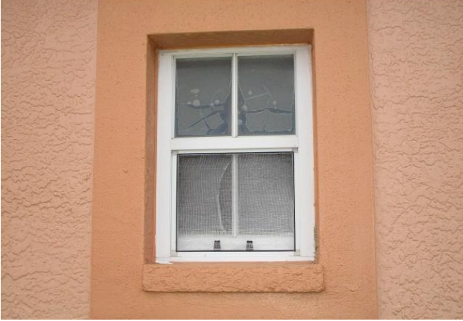
#7) opening protection: non impact windows
