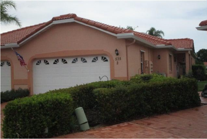
#5) roof geometry: "other" style roof **wall type construction: 85% reinforced masonry
