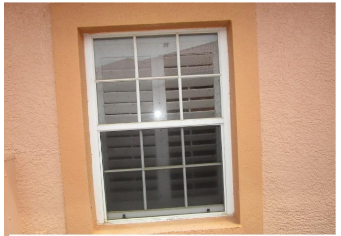
#7) opening protection: non impact windows
