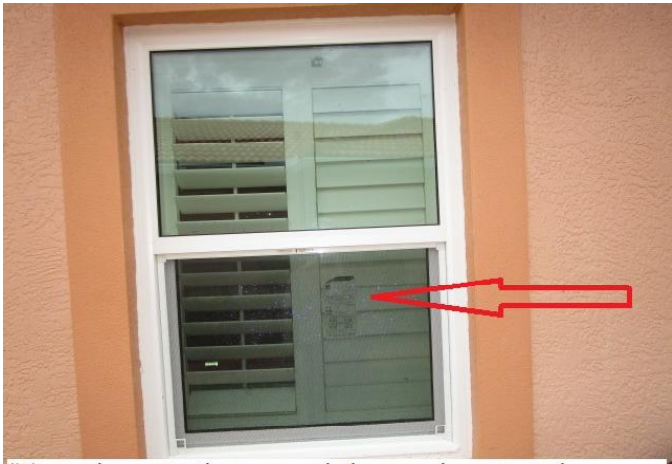
#7) opening protection: some windows are impact rated
