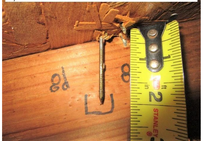
#3) roof deck attachment: 8d nails
