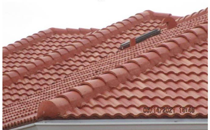
#2) roof covering: 2020 TILE HIP style roof PRBD2020-0731307 applied 7/31/2020
