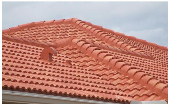
#2) roof covering: 2020 TILE HIP style roof PRBD2020-0731283 applied 7/31/2020
