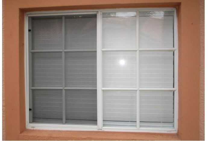
#7) opening protection: non impact windows
