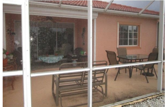
#7) opening protection: non impact rear sliders w/storm fabric or roll down shutters
