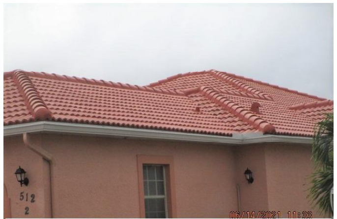
#2) roof covering: 2020 TILE HIP style roof PRBD2020-0731278 applied 7/31/2020
