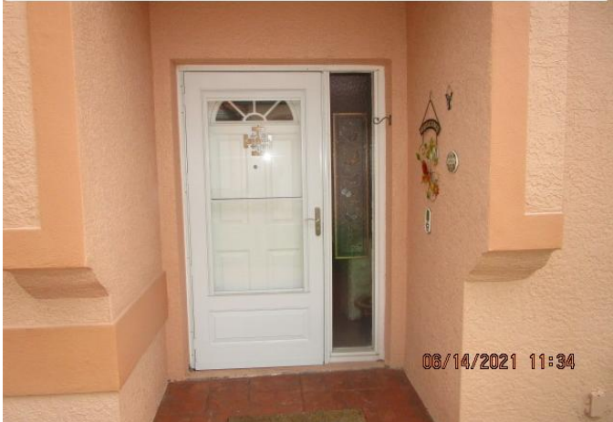
#7) opening protection: non impact front entrances
