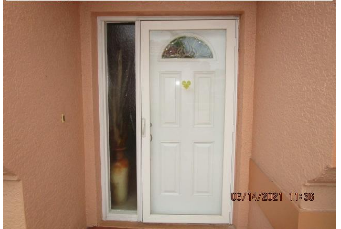
#7) opening protection: non impact front entrances
