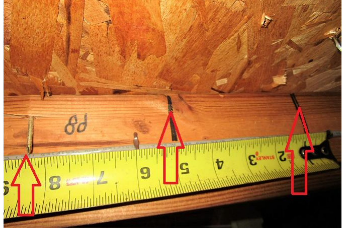
#3) roof deck attachment: 8d nail spacing
