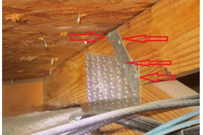
#4) roof to wall attachment: single wrap- opposite view
