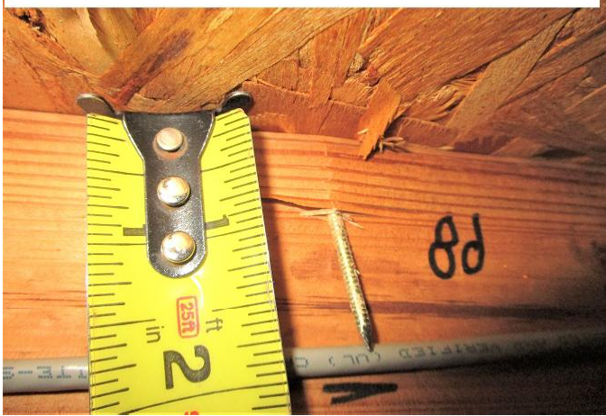
#3) roof deck attachment: 8d nails
