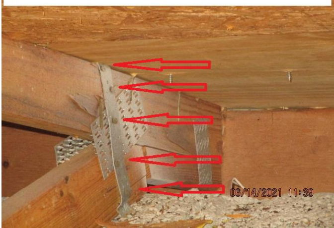
#4) roof to wall attachment: single wraps- front view
