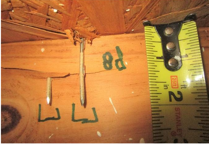
#3) roof deck attachment: 8d nails
