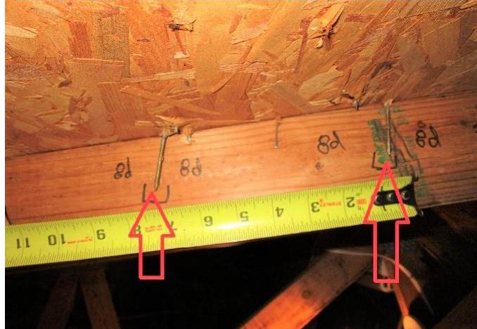
#3) roof deck attachment: 8d nail spacing
