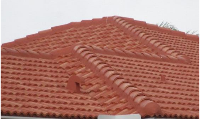
#2) roof covering: 2020 TILE HIP style roof PRBD2020-0731312 applied 7/31/2020
