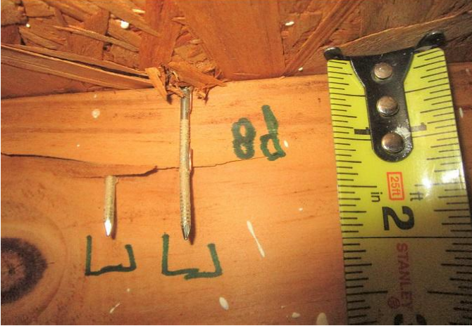
#3) roof deck attachment: 8d nails
