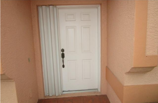
#7) opening protection: non impact front entrances w/panels or shutters
