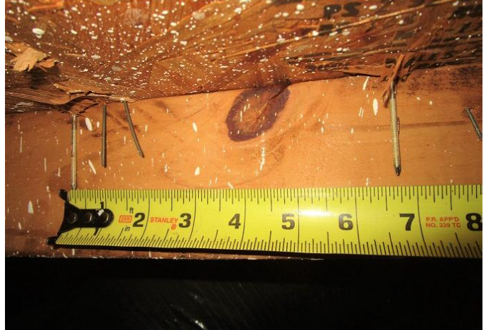
#3) roof deck attachment: 8d nail spacing
