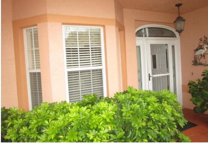
#7) opening protection: non impact windows
