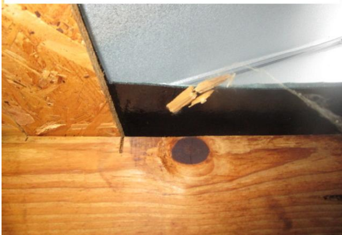
#6) secondary water barrier as viewed from the attic
