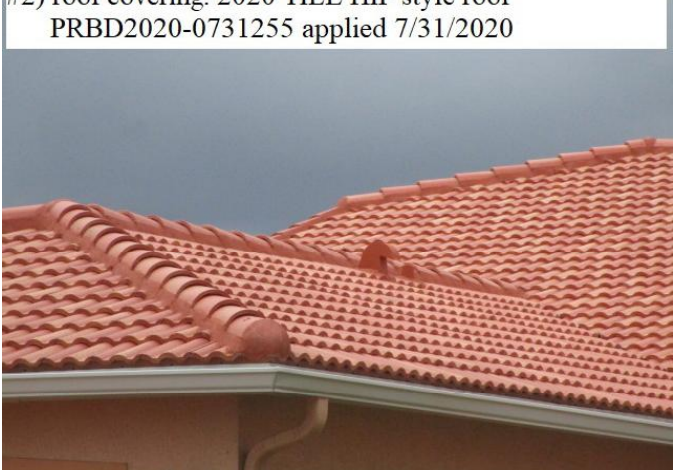
#2) roof covering: 2020 TILE HIP style roof
