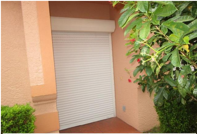
#7) opening protection: metal clad door w/accordion shutters or roll down shutters
