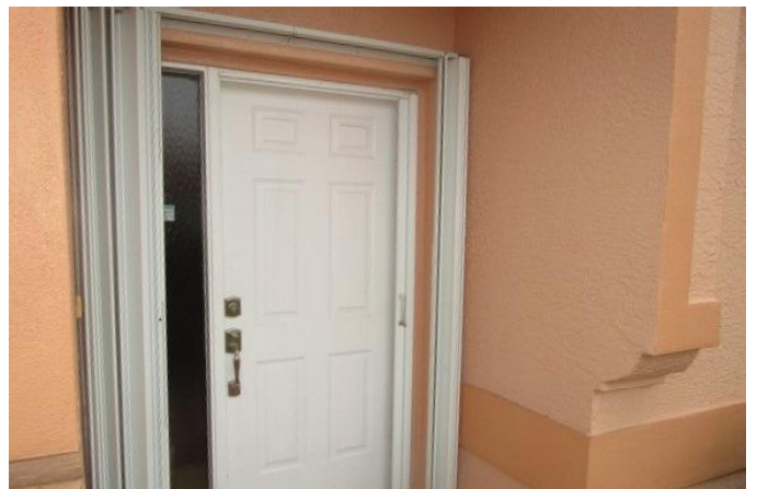
#7) opening protection: metal clad door w/accordion shutters or roll down shutters
