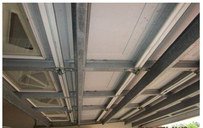
#7) opening protection: wind rated non impact garage doors
