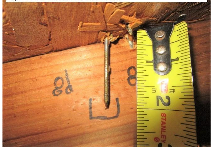
#3) roof deck attachment: 8d nails
