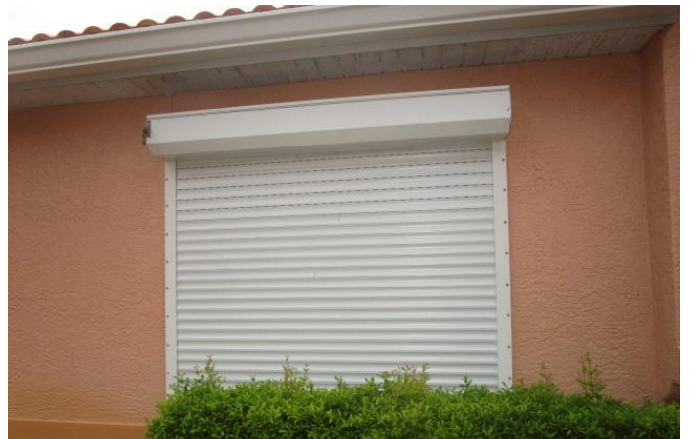
#7) opening protection: non impact windows, doors & sliders all with some form of protection (metal panels or roll downs)
