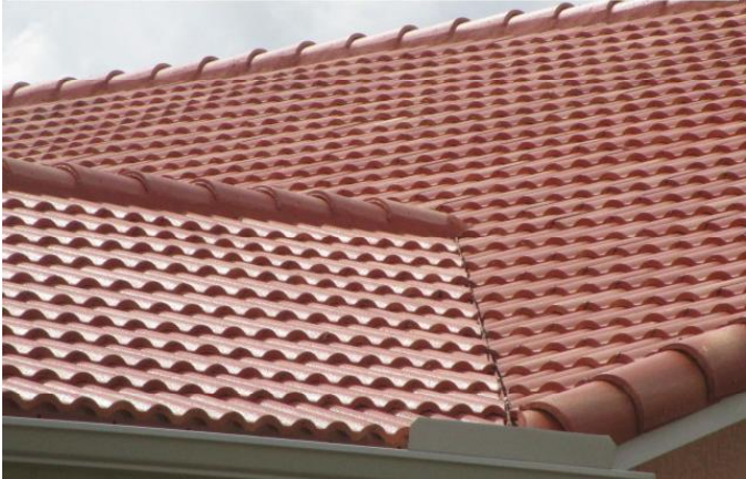
#2) roof covering: 2020 TILE HIP style roof PRBD2020-0731257 applied 7/31/2020
