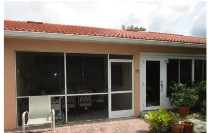
#7) opening protection: non impact rear sliders some w/protection some without protection
