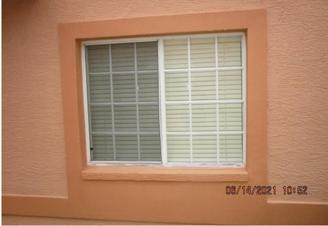
#7) opening protection: non impact windows
