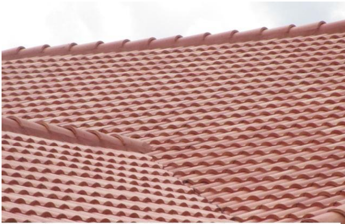
#2) roof covering: 2020 TILE HIP style roof PRBD2020-0731317 applied 7/31/2020
