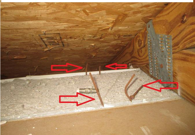
***wall type construction: 85% reinforced masonry
