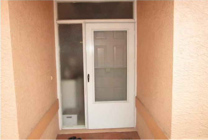
#7) opening protection: metal clad door w/non impact transom & sidelite windows
