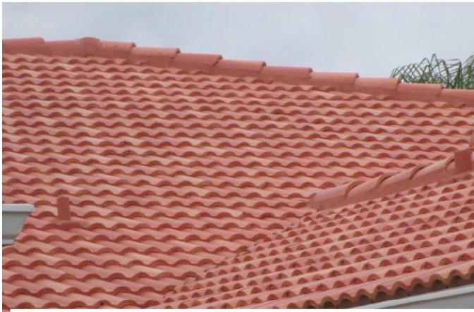
2) roof covering: 2020 TILE HIP style roof PRBD2020-0731319 applied 7/31/2020
