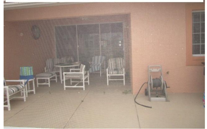
#7) opening protection: lanai- non impact sliders *one w/roll down shutters
