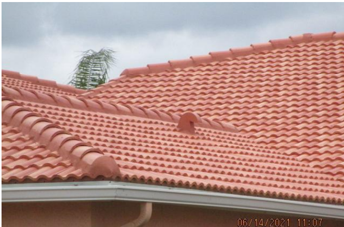
#2) roof covering; 2020 TILE HIP style roof PRBD2020-0731321 applied 7/31/2020
