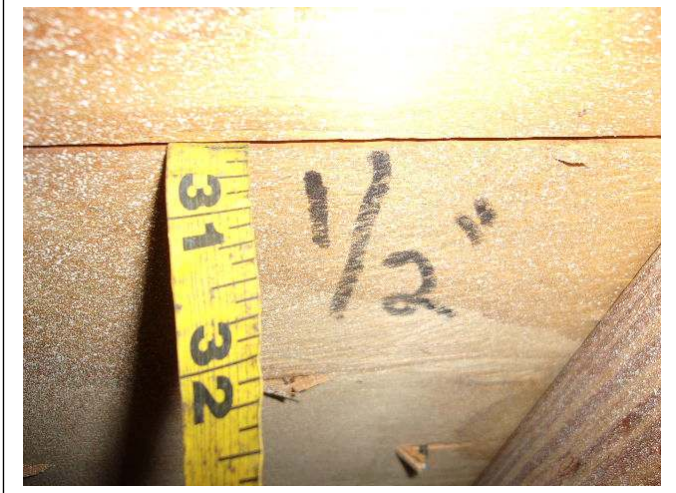
ROOF DECK THICKNESS – ½ inch plywood
