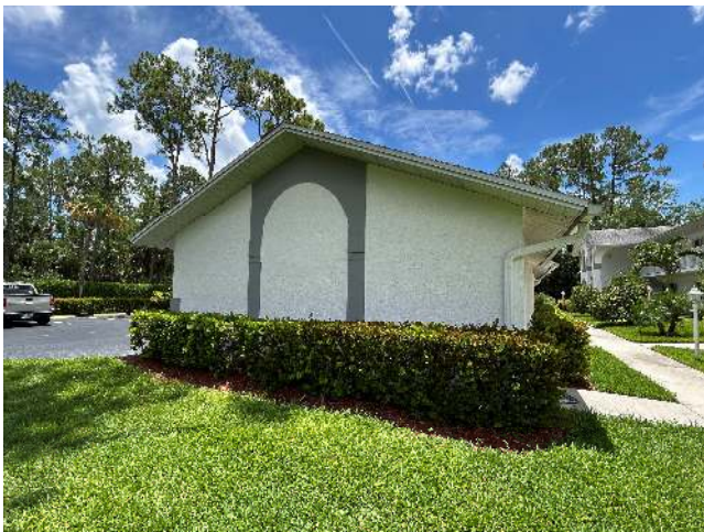
ROOF GEOMETRY – Gable / Other Roof Shape
