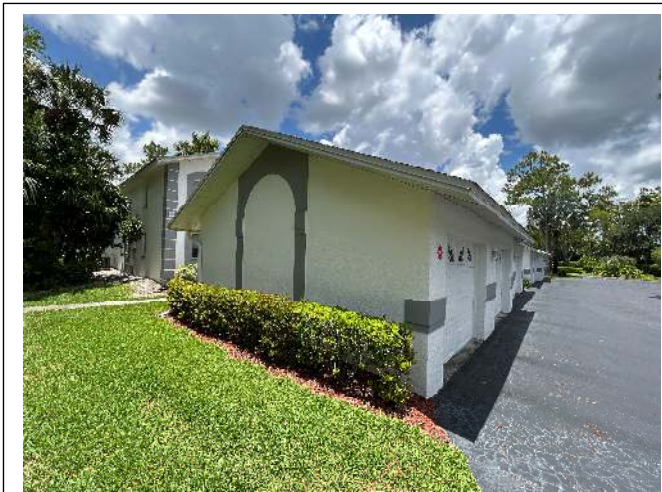
ROOF GEOMETRY – Gable / Other Roof Shape
