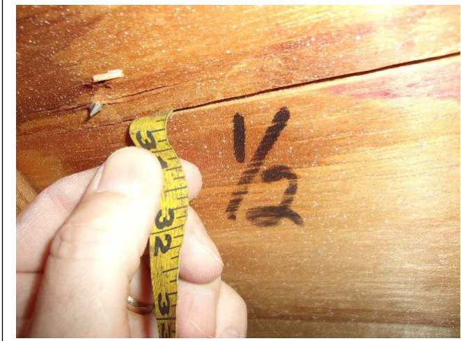
ROOF DECK THICKNESS – ½ inch plywood
