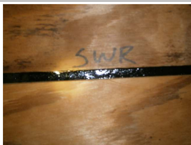
SECONDARY WATER BARRIER – A polymer adhesive (peel & stick) SWR Barrier was installed on the entire roof deck in 2018
