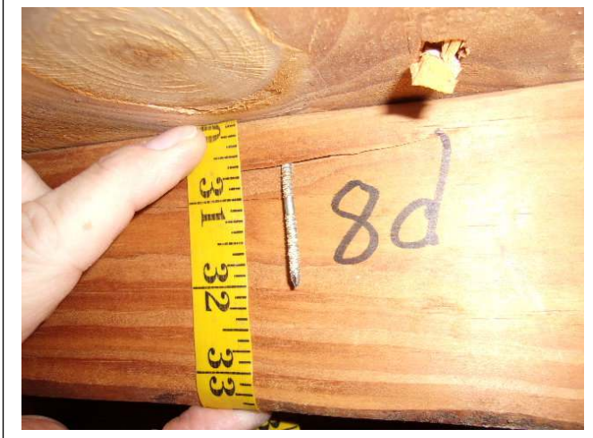
ROOF DECK ATTACHEMNT – 8d ring shank nails added in 2018
