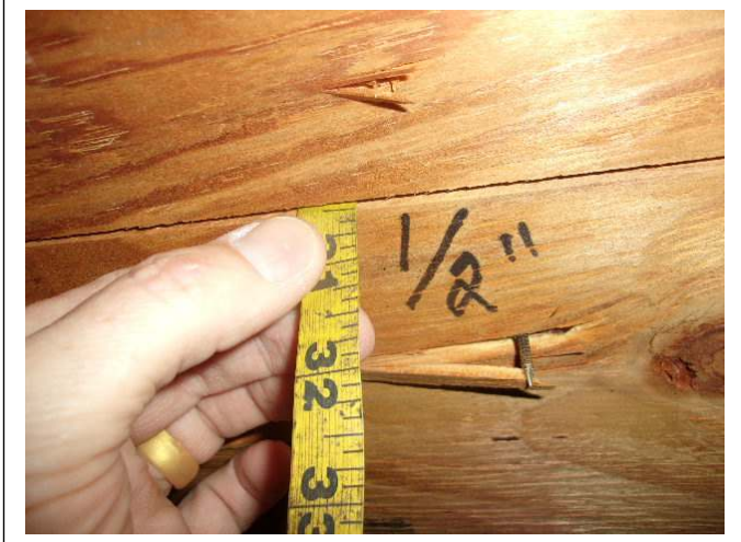
ROOF DECK THICKNESS – 1/2 inch plywood
