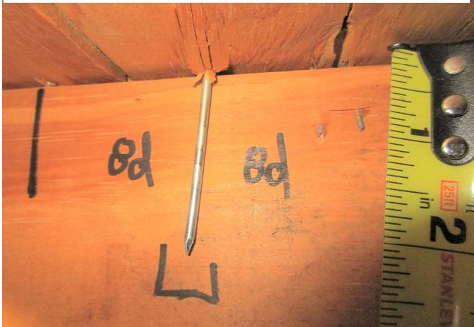
#3) roof deck attachment: 8d nails
