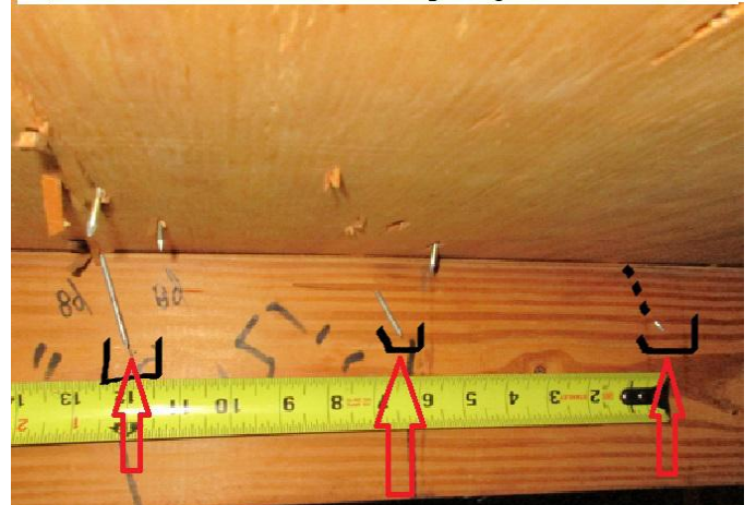
#3) roof deck attachment: 8d nail spacing
