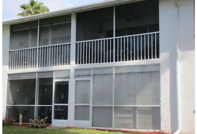
#7) opening protection: non impact sliders (some w/shutters)
