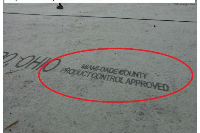
#6) secondary water barrier
