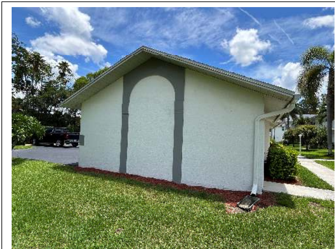
ROOF GEOMETRY – Gable / Other Roof Shape
