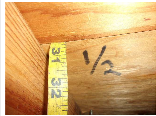
ROOF DECK THICKNESS – 1/2 inch plywood
