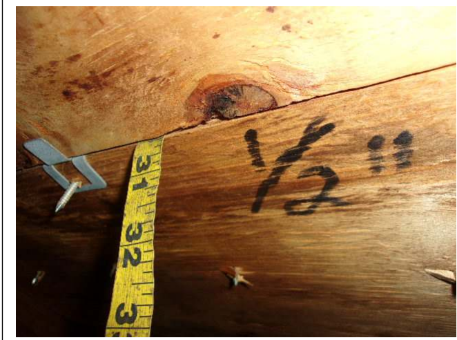
ROOF DECK THICKNESS – ½ inch plywood
