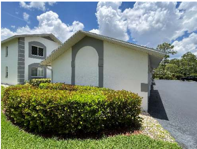
ROOF GEOMETRY – Gable / Other Roof Shape
