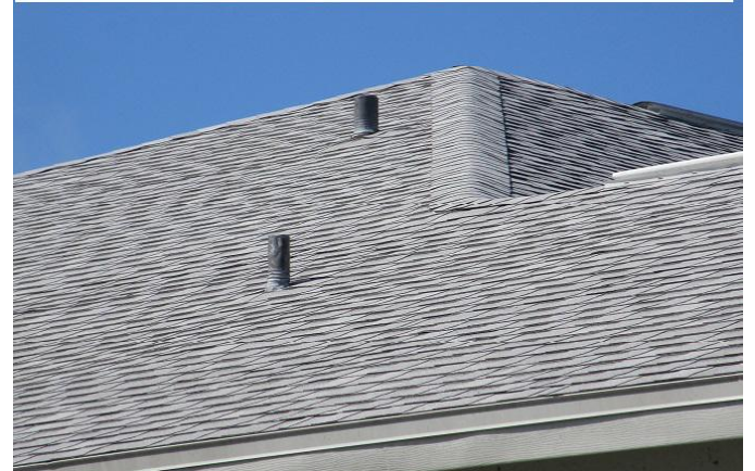
#2) roof covering: 2018 dimensional asphalt shingle HIP style roof PRBD2018-0848384 applied 8/13/2018
