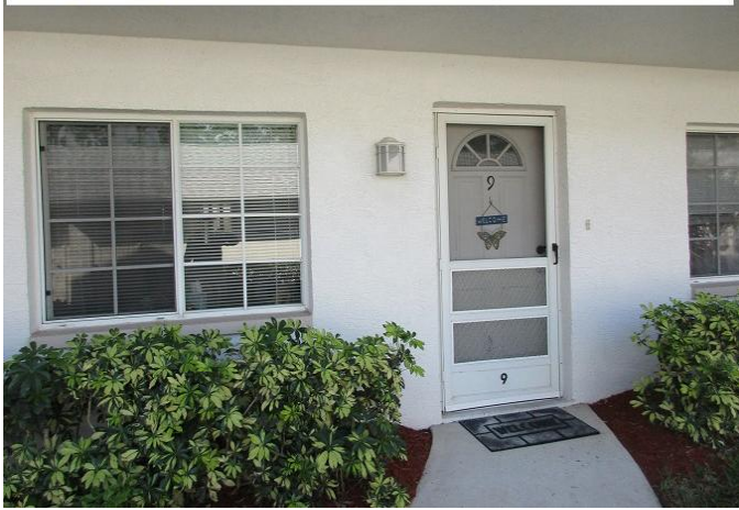
#7) opening protection: non impact front entrance
