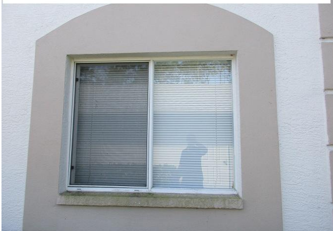
#7) opening protection: non impact windows
