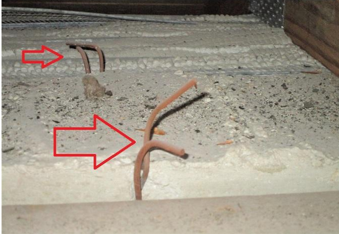
**wall type construction: 90% reinforced masonry
