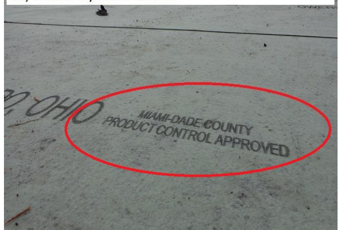
#6) secondary water barrier
