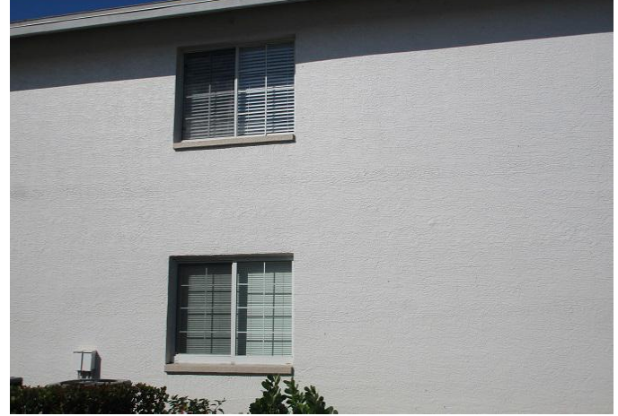
#7) opening protection: non impact windows
