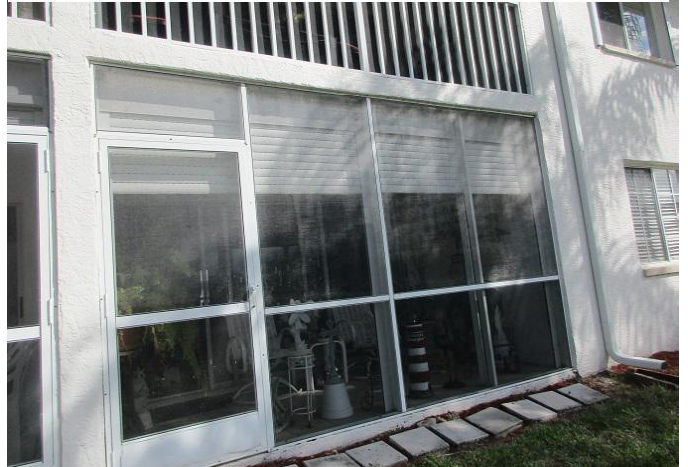
#7) opening protection: non impact sliders some w/shutters
