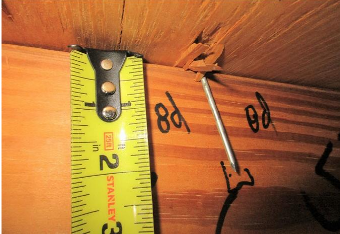
#3) roof deck attachment: 8d nails
