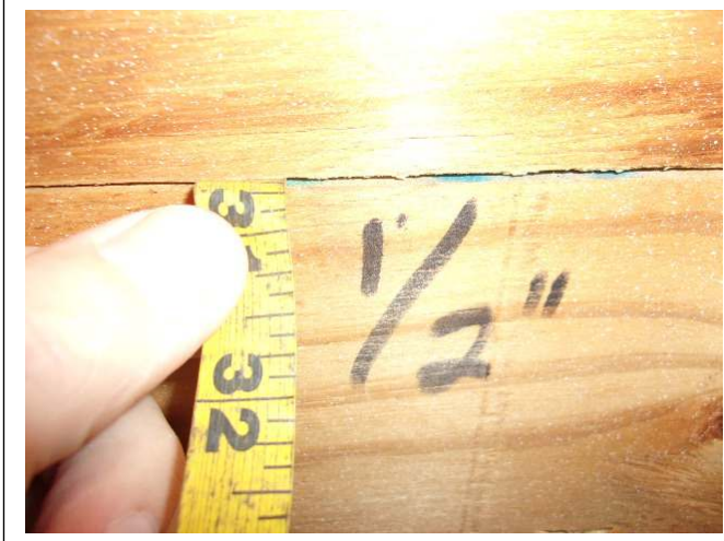
ROOF DECK THICKNESS – ½ inch plywood
