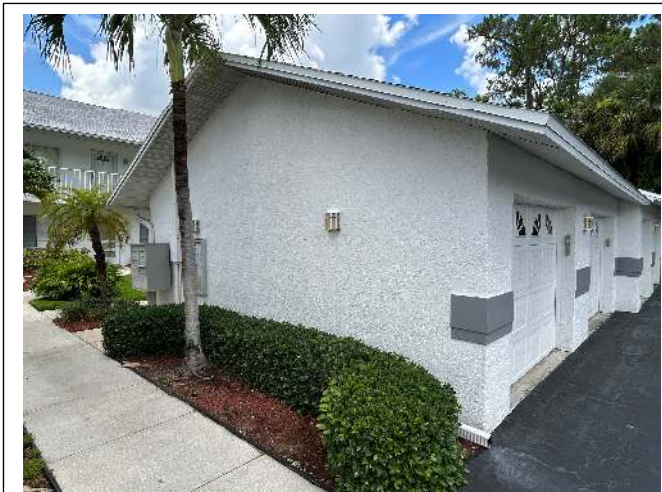
ROOF GEOMETRY – Gable / Other Roof Shape
