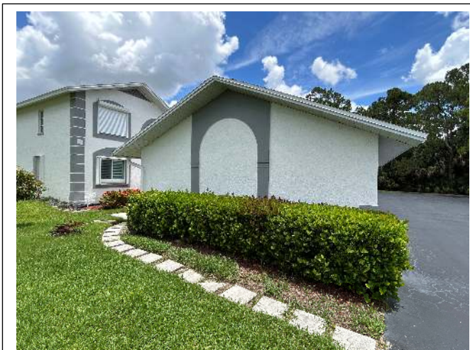
ROOF GEOMETRY – Gable / Other Roof Shape
