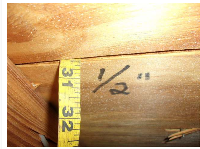
ROOF DECK THICKNESS – ½ inch plywood
