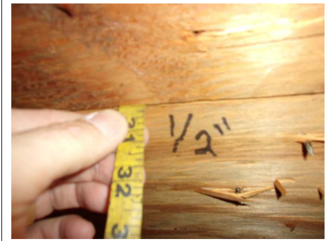
ROOF DECK THICKNESS – 1/2 inch plywood
