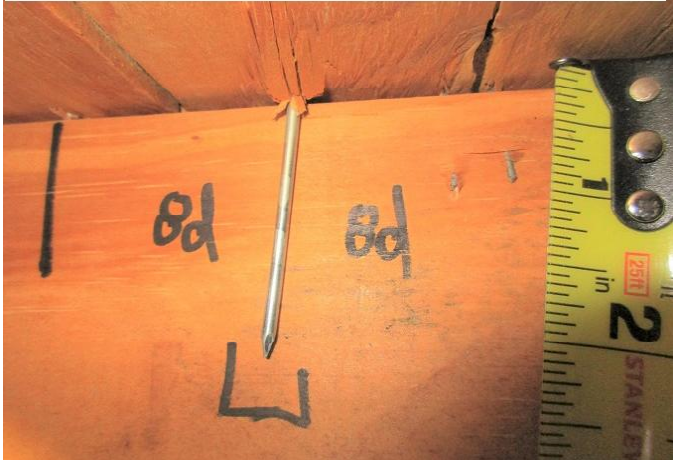
#3) roof deck attachment: 8d nails
