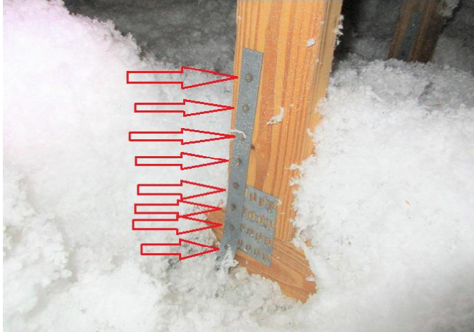
#4) roof to wall attachment: hurricane clips
