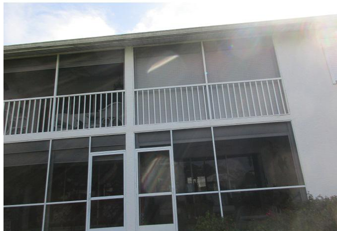
#7) opening protection: non impact sliders (some w/shutters)
