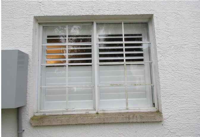
#7) opening protection: non impact windows
