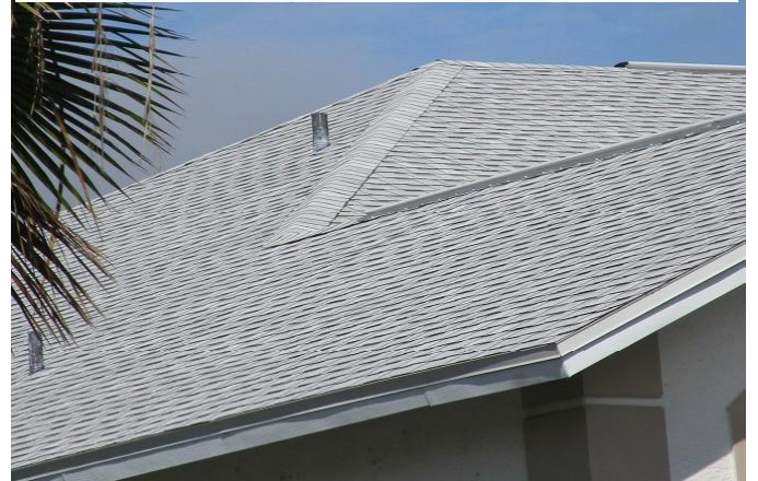
#2) roof covering: 2018 dimensional asphalt shingle HIP style roof PRBD2018-0848390 applied 8/13/2018
