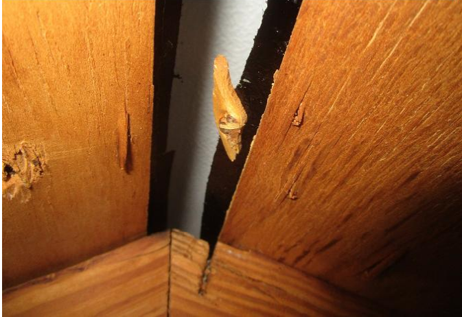
#6) secondary water barrier/resistance as viewed from the attic
