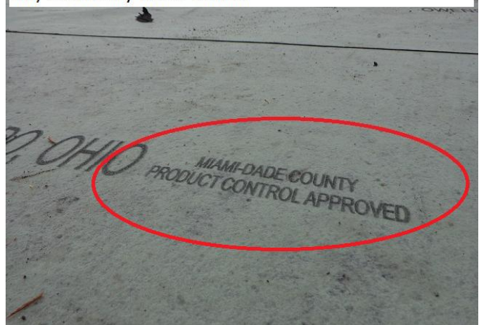
#6) secondary water barrier
