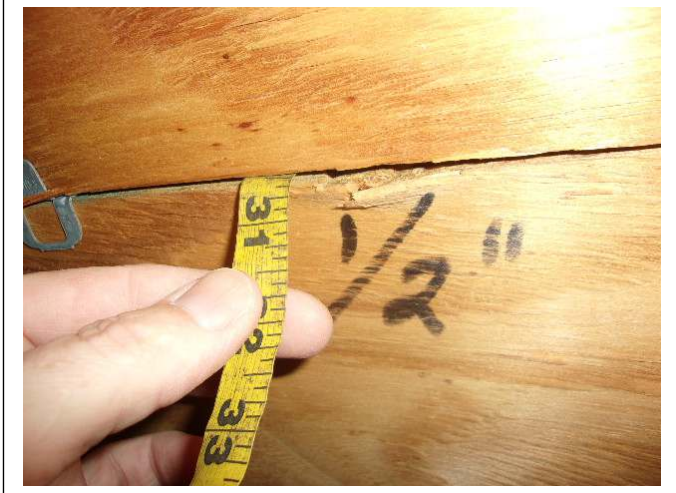
ROOF DECK THICKNESS – ½ inch plywood
