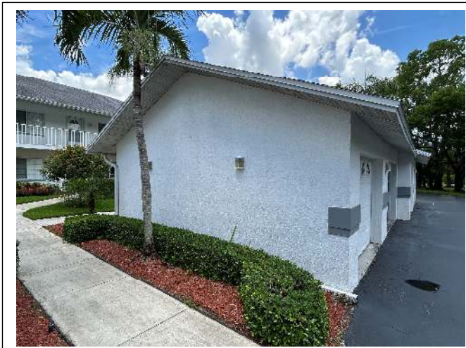
ROOF GEOMETRY – Gable / Other Roof Shape
